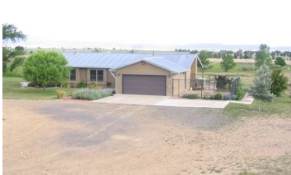
4 car concrete parking
